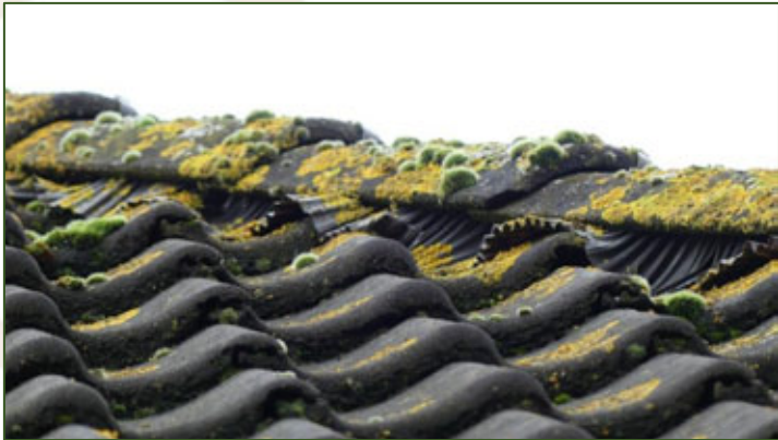
Openingen dakpannen, boerderij (bron: FF Solutions)
