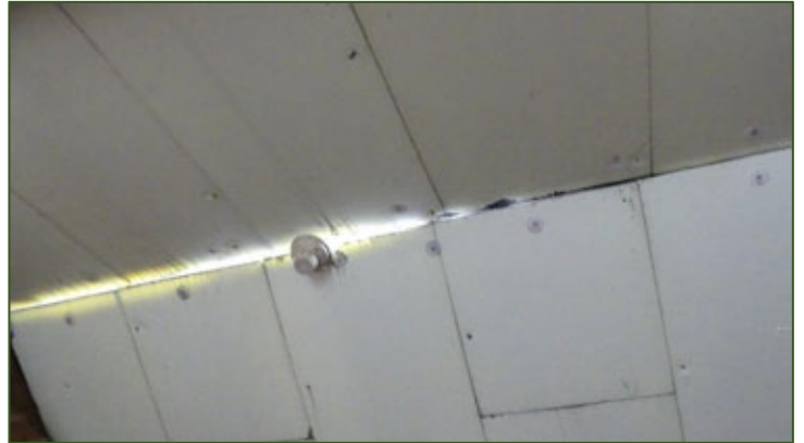
Openingen dak opstal C (bron: FF Solutions)
