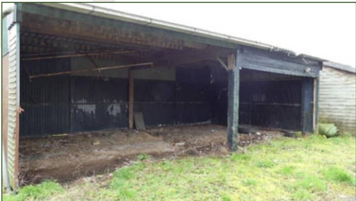
Overkapping, opstal D (bron: FF Solutions)
