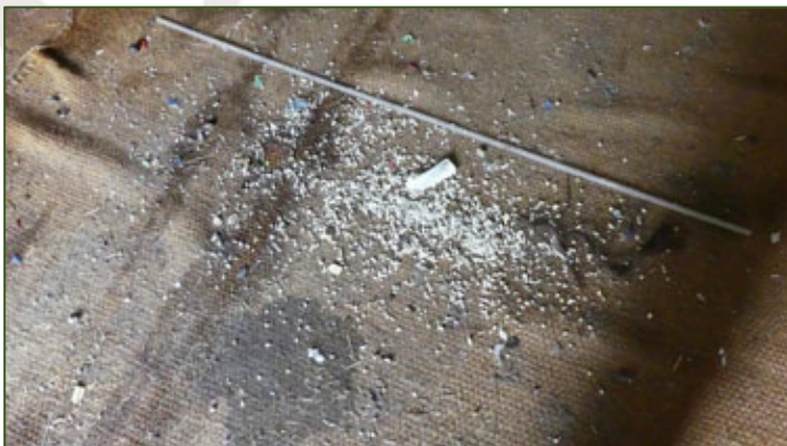
Resten dakisolatie, sporen o.a. steenuil (bron: FF Solutions)
