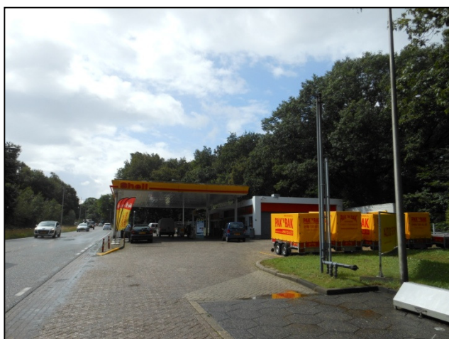
Foto 3: Tankstation, Daam Fockemalaan 18
